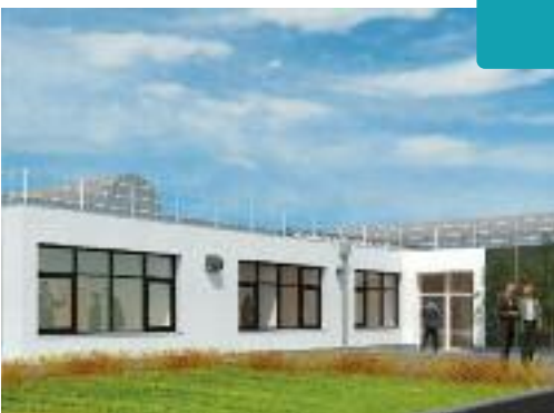
CENTRE TECHNIQUE MUNICIPAL.
